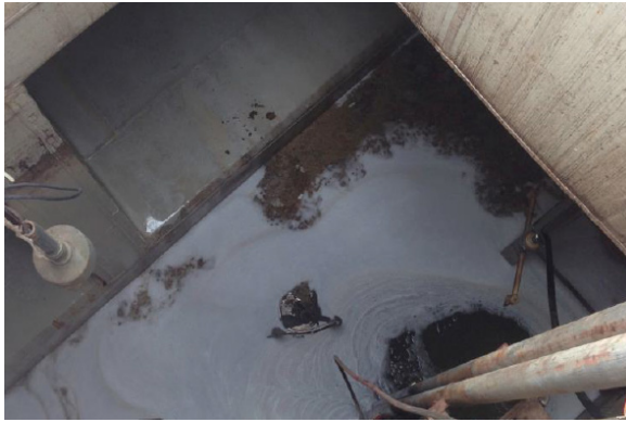
Accelerating Breakdown of Grease Cap
