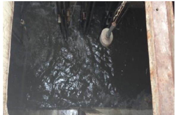
With Air Blower No Grease Caps Remaining
