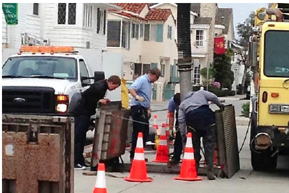
Vacuum Cleaning of Pump Station
