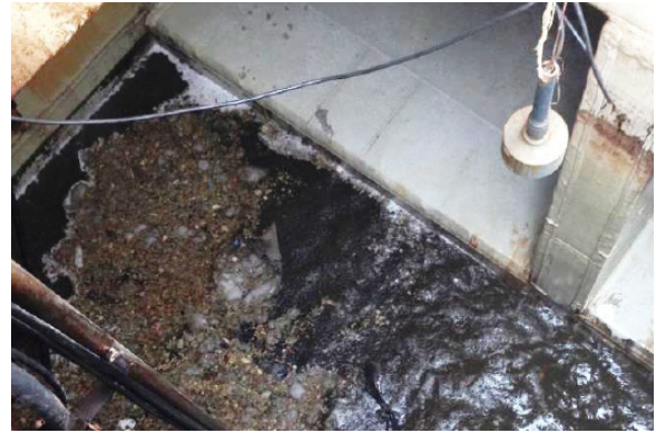
Highly Degraded Floating Grease Cap
