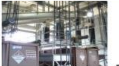
ODOR CONTROL FOR THE GRIT SCREENING CONVEYOR OPERATION MISSISSAUGA WWTP, CANADA
