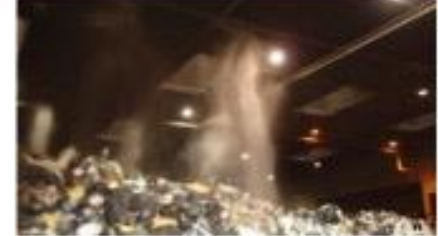
BOC ODOR CONTROL USING MISTING SYSTEM
