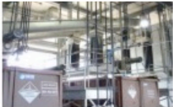
ODOR CONTROL FOR THE GRIT SCREENING CONVEYOR OPERATION MISSISSAUGA WWTP, CANADA
