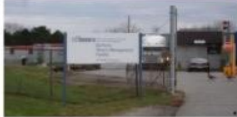
WASTE TRANSFER STATIONS TORONTO, CANADA
