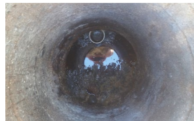
Drain cleaned with Eco-Cat Clean™
