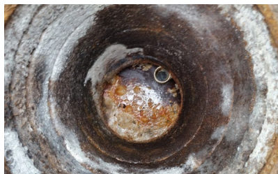
Drain cleaned with a bacterial/enzyme product
