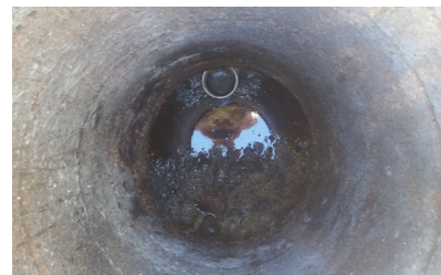
Drain cleaned with Eco-Cat Clean™
