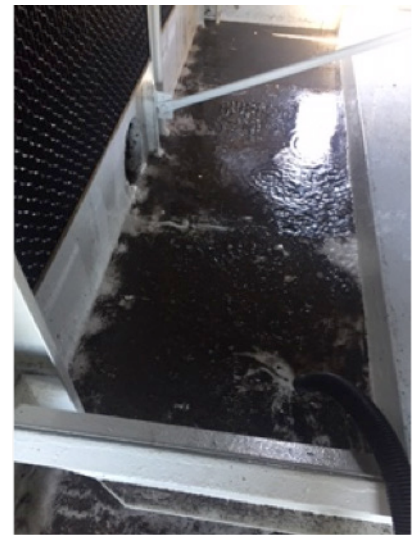
Figure 3 Top: Typical Organic Sump contamination Below: Contamination after BOC treatment
