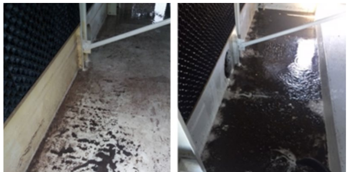
Typical Organic Sump contamination on the right, contamination after BOC treatment.
