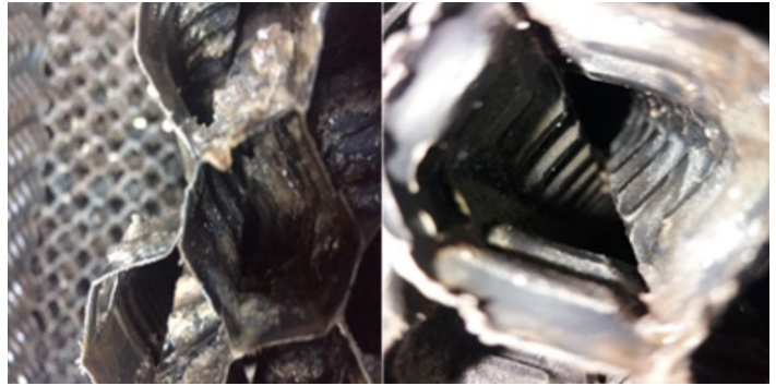
Fill pack before and after, notice the absence of biofilm on the after picture.
