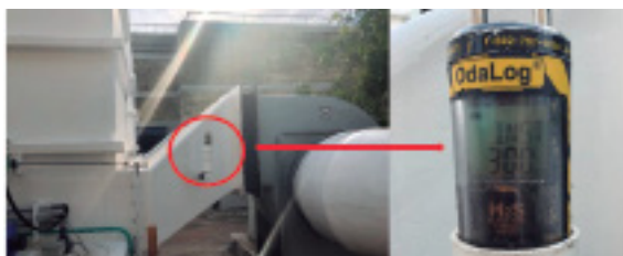
FIGURE 4. Scrubber entry (left) and measurement of H 2 S with OdaLog equipment.
