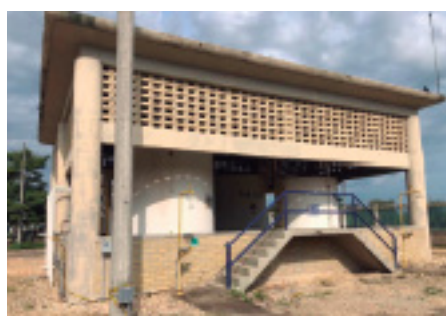
FIGURE 2. Storage tanks for conventional chemistry product.
