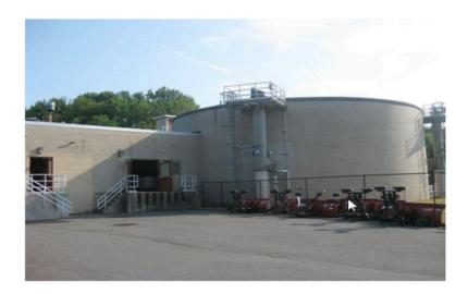
2-AS's operated as complete mix, **mesophilic**, with primary and was sludge and FOG's. With 1 Primary and 1 secondary AD (500,000 gal./AD).
