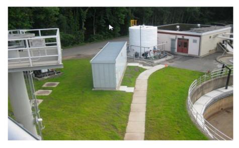
FOG receiving began operation in Feb, 2013. Original design was 11,000 Gallon, which has been expanded to 30,000 gallons, with automatic mixing and temperature control.
