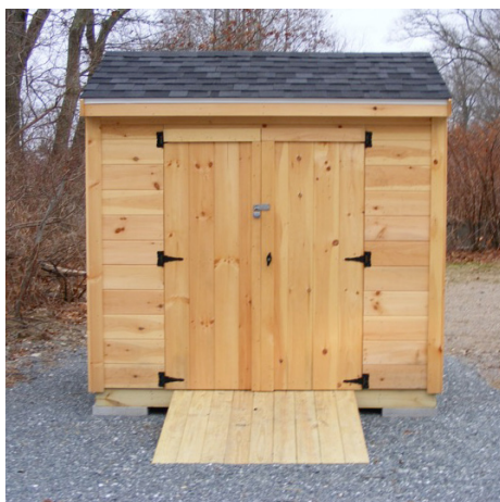
Sewer Odor Control Shed
