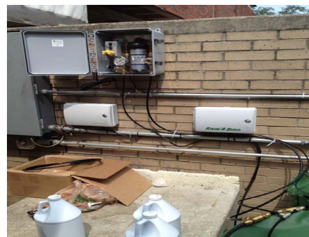
Master Panel For 4 spray heads
