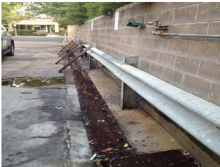
One Spray Head For Leach Drain Odors
