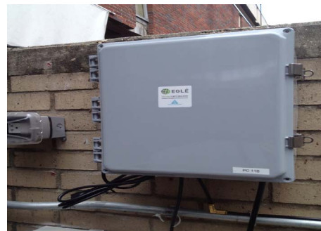
Master Panel For 4 spray heads
