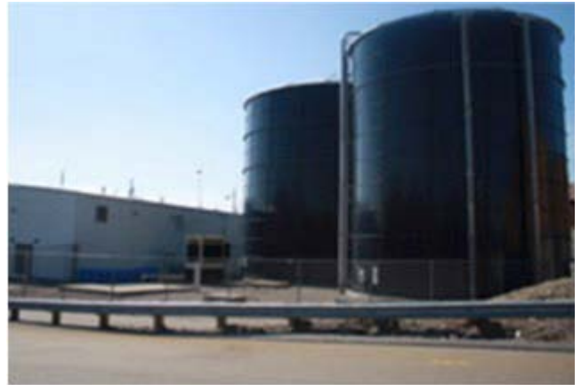
WWTP and E.Q. Tanks
