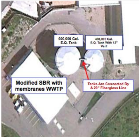
WWTP and E.Q. Tanks
