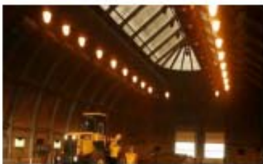
ODOR CONTROL IN NEW YORK CITY- RESIDUAL WASTE FACILITY- (COMBINATION OF GRIT SCREENING AND FOG'S )
